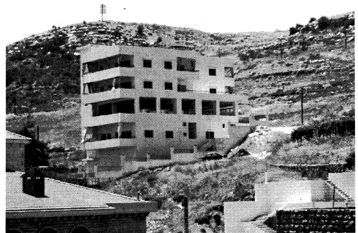
Fig. 6. Shanay, Lebanon: typical rural residential development following the Building Law specifications: note the pilotis ground floor.
