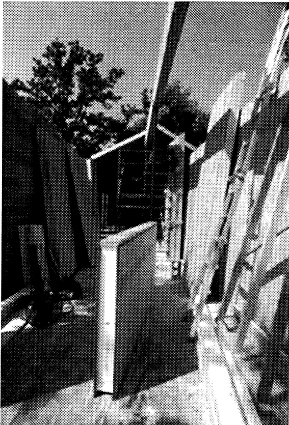
Fig. 2 Photo describing the use of modular materials that determined the length, width and breadth of the house as it fit into the narrow site conditions. Structurally insulated panels were used to test and confirm the added benefits of thermal control of this product. The SIS used materials that offered an option to traditional, stick built construction methods.
