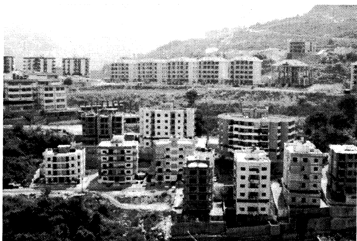
Fig. 1. Bsalim, Lebanon: new suburban developments that show the way the landscape is flattened to accommodate residential block in accordance with legal specifications.
