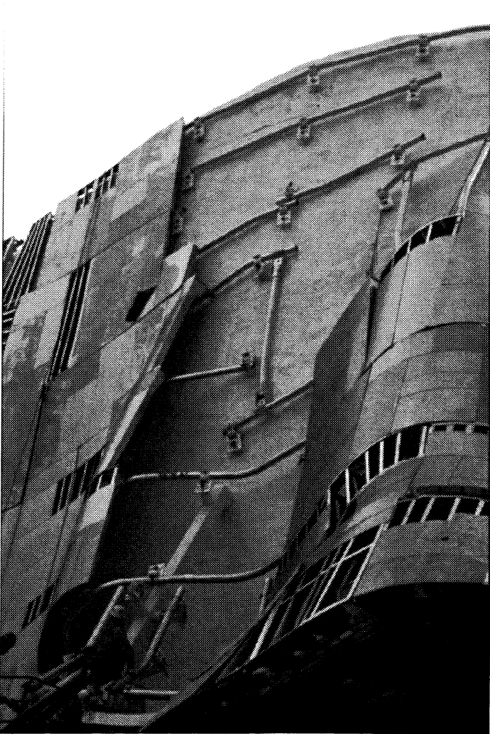
Fig. 1. EMP under construction.
