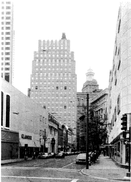
Fig. 7. View of Carondelet Street from Canal Street showing American Bank Building. Nathaniel Curtis for Moise H. Goldstein. 1928-29 (left of center) and Hibernia Bank Tower. Favrot & Livaudais. 1919 (cupola right of center).
