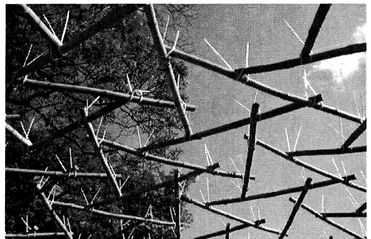
Figure 10: View of bamboo structure from inside
