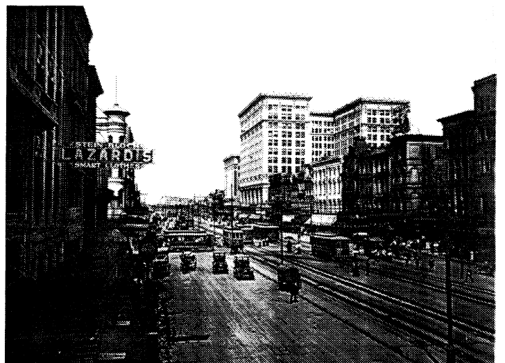
Fig. 5. Canal Street. c. 1910. Detroit Publishing Co., Courtesy Library of Congress.
