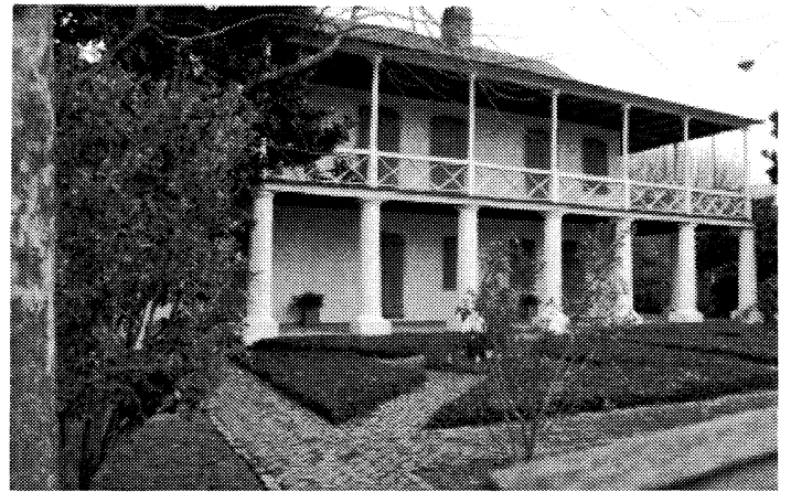
Fig. 4. Pitot House. 1796-99. View from Bayou St. John.
