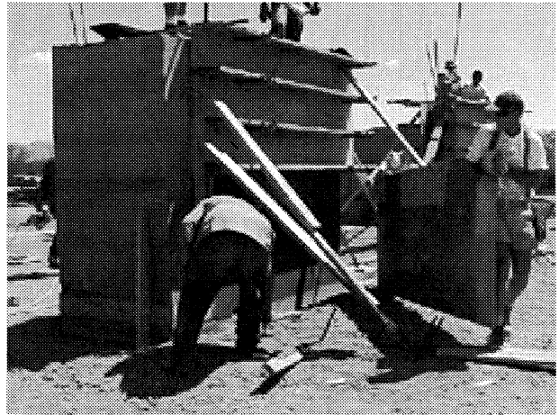
Stripping forms from Gila house.
